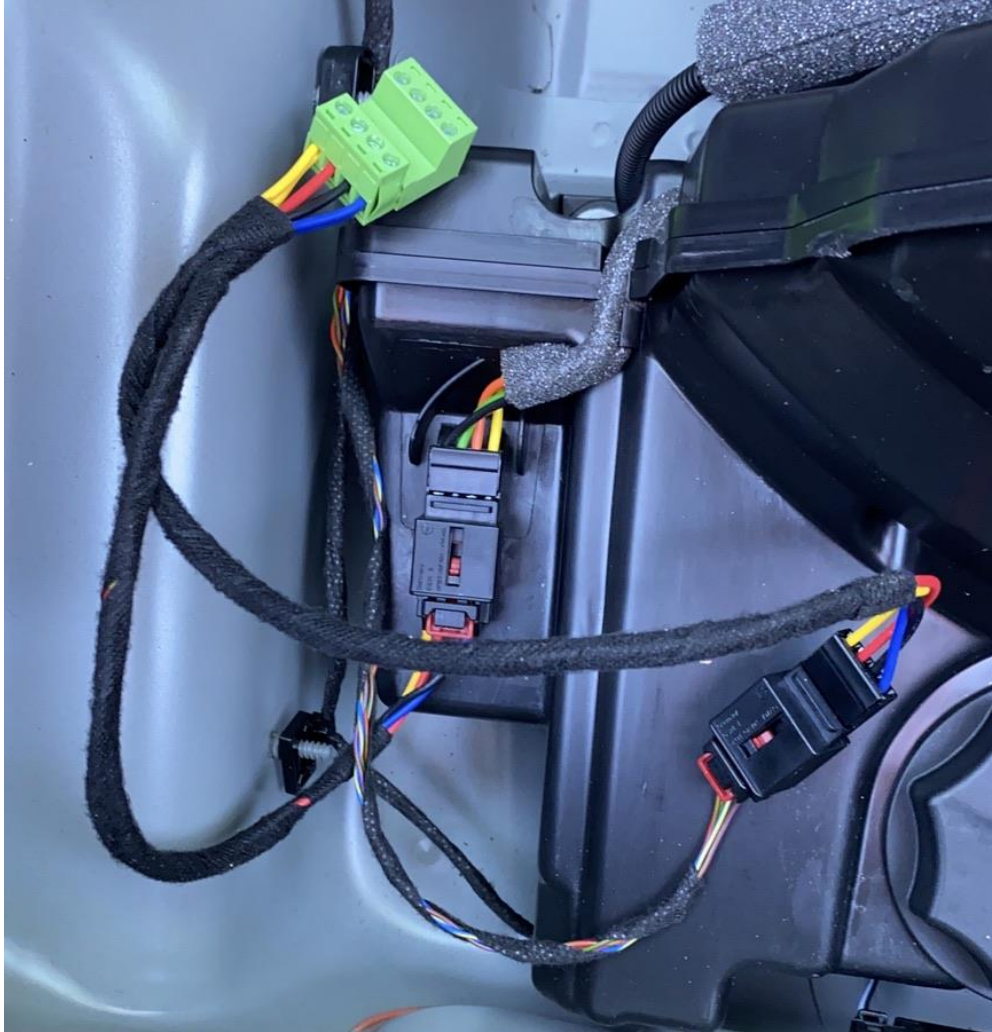
Figure 11: Bruce's cable plugged between car's wiring harness and OEM subwoofer.
