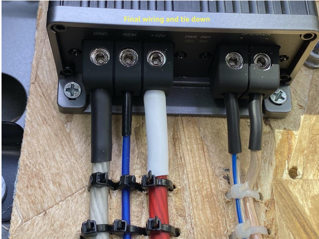
Figure 24: Final Wiring and Tie Down
